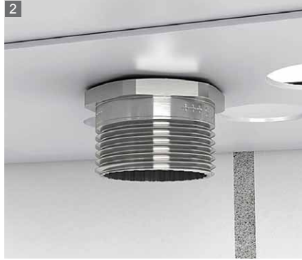
2 Install the connector onto the enclosure.
